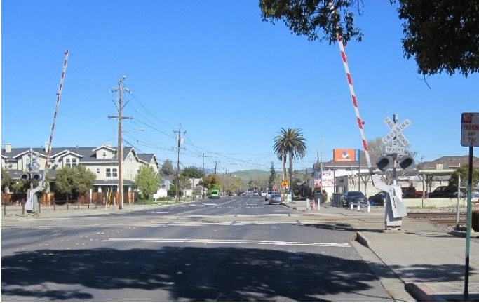
A typical at-grade crossing that requires improvement. This location is at L Street in the City of Livermore.
