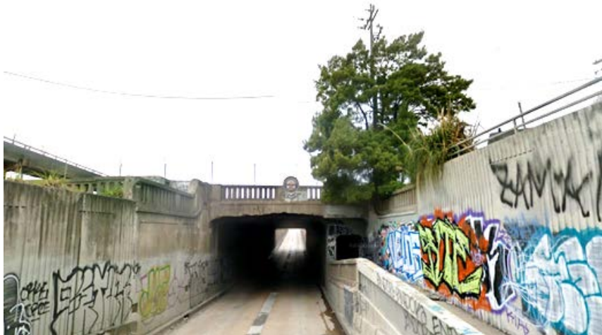
7th Street, approaching Union Pacific Railroad bridge from the east.
