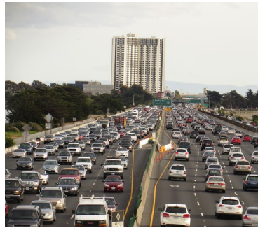
I-80 freeway looking south approaching the Ashby Avenue exit.
