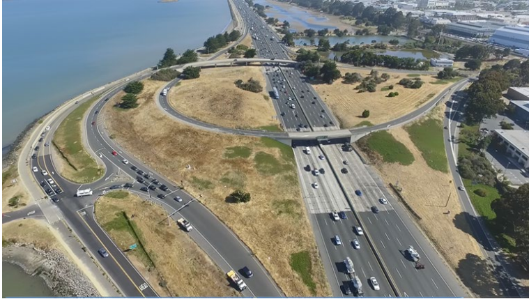
Aerial view of I-80/Ashby Avenue (SR-13) interchange.
