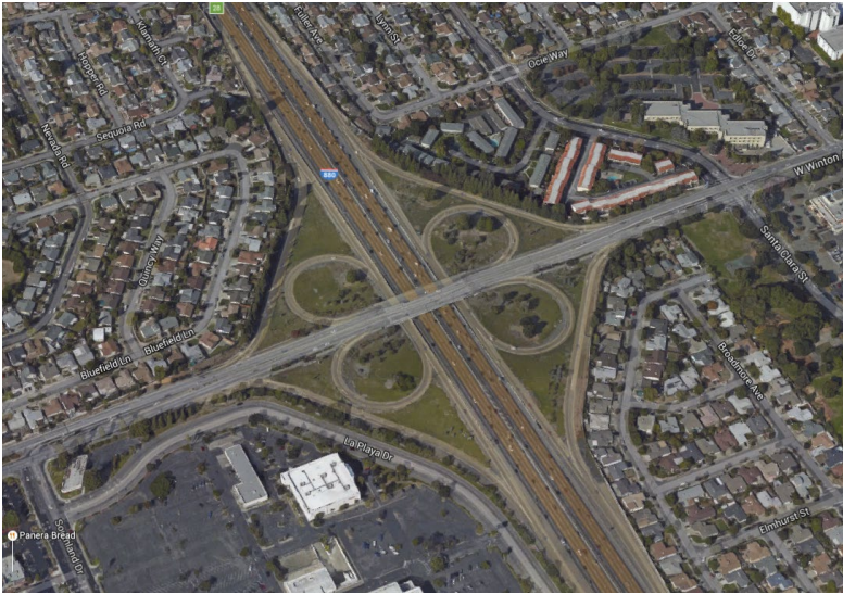
Current interchange at I-880/Winton Avenue.
