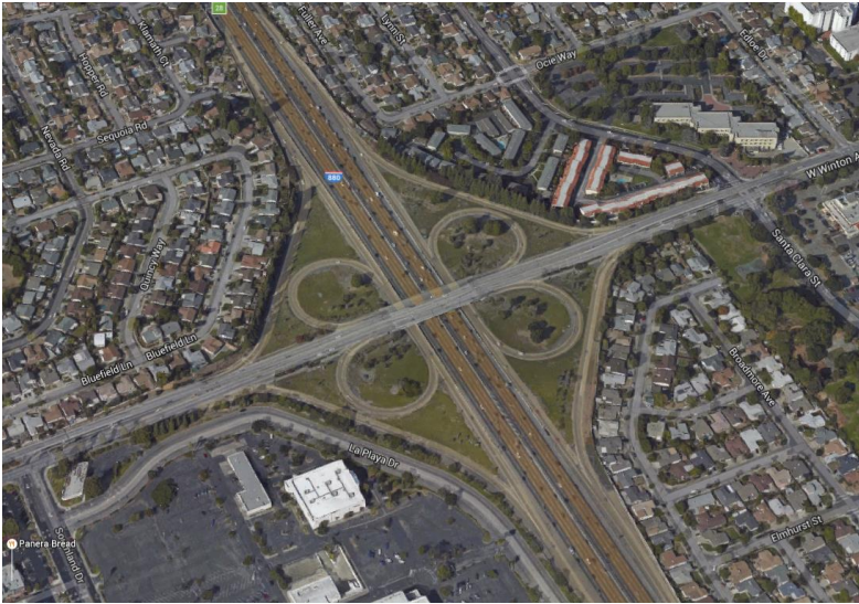
Current interchange at I-880/Winton Avenue.
