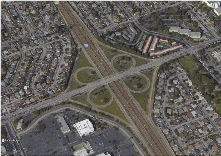
Current interchange at I-880/Winton Avenue.
