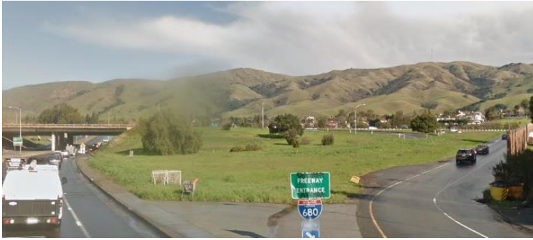
Eastbound SR-262 at the I-680 southbound on-ramp.
