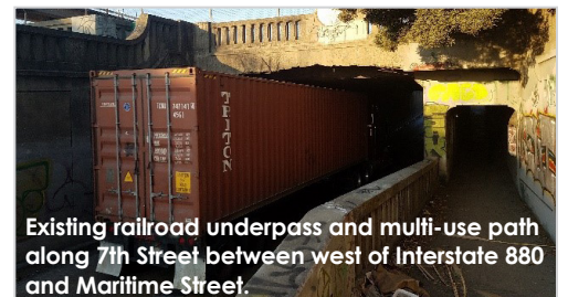
Existing railroad underpass and multi-use path along 7th Street between west of Interstate 880 and Maritime Street. Project Updates cont'd on page 2
