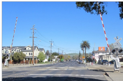
A typical at-grade crossing at L Street in the City of Livermore that requires improvement.
