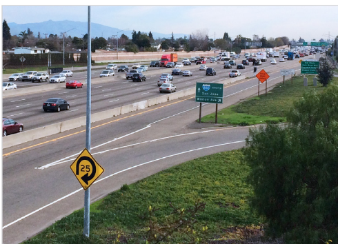
Winton Avenue off-ramp facing southbound on Interstate 880.
