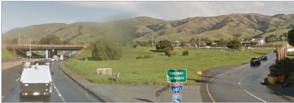
Facing eastbound on State Route 262 at the Interstate 680 on-ramp.
