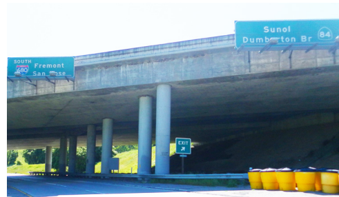
Interstate 680 southbound toward Sunol near the State Route 84 interchange.
