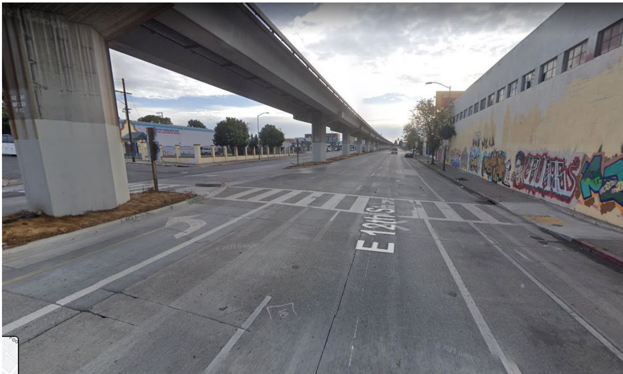
H-7 | E12 th Street at 22nd Avenue in Oakland: Bike lanes are discontinuous & require cyclists to weave across multiple lanes to make left turns
