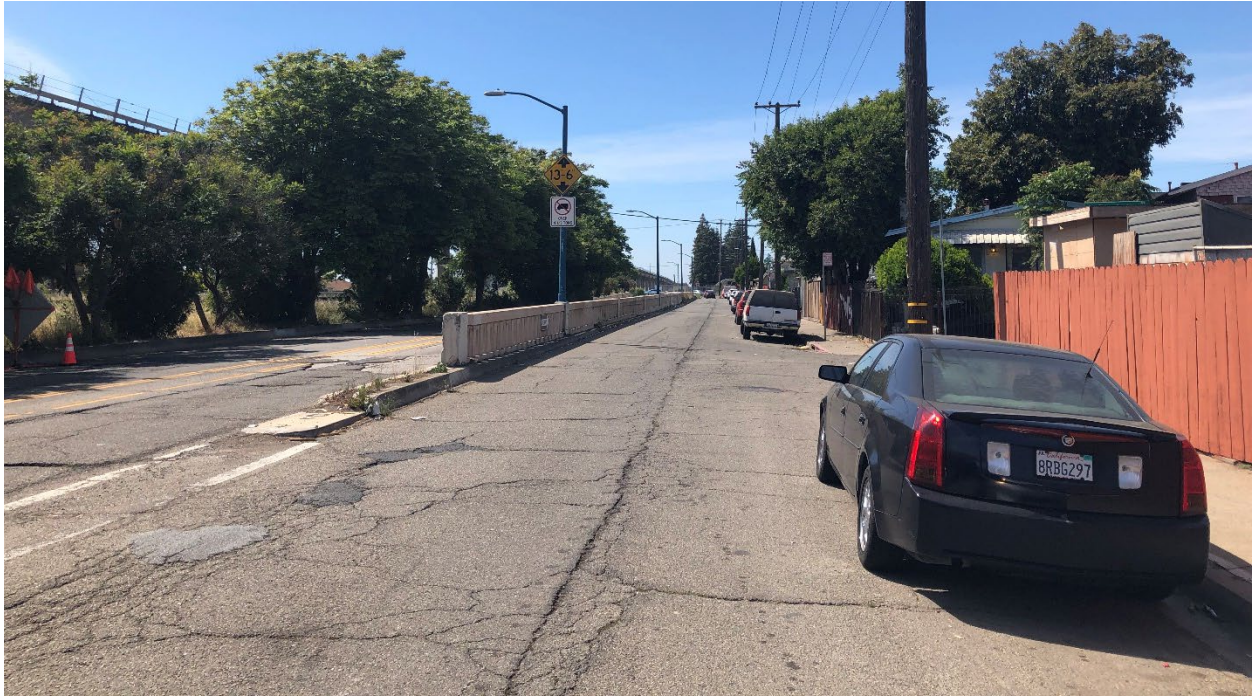
H-18 | San Leandro Street at Blenheim Street in Oakland: Narrow pavement widths do not allow for safe passing of bicyclists
