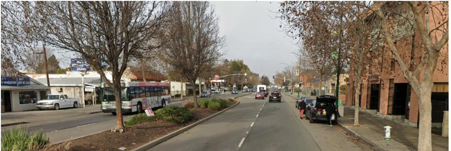
East 14th Street in Alameda County.
