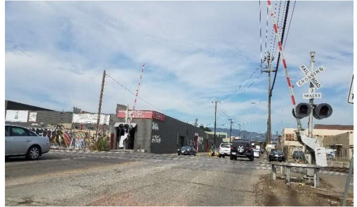
Northeast approach to the rail crossing along High Street in the City of Oakland.
