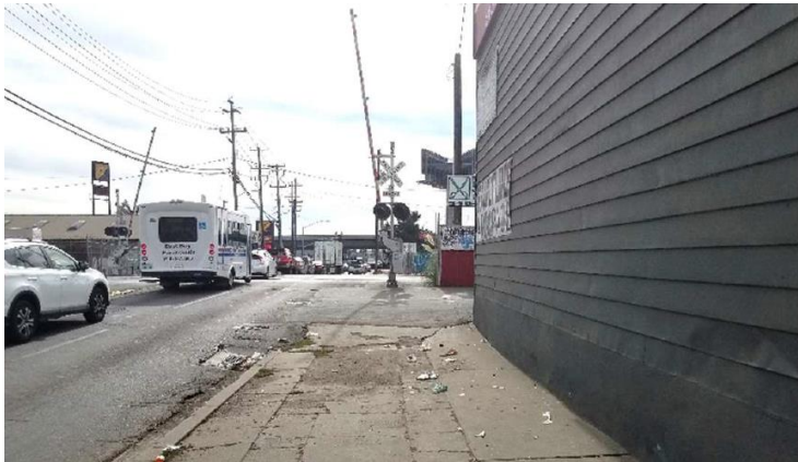
Southwest approach to the rail crossing along High Street in the City of Oakland.
