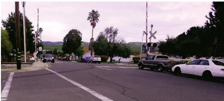
Northbound approach to the rail crossing on H Street in Union City.
