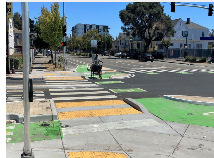
Protected Intersection at West St & W MacArthur Blvd
