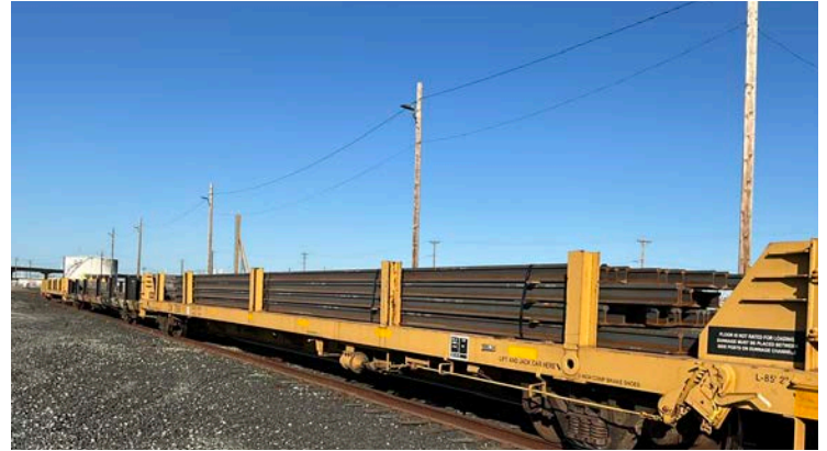
New rail being delivered to the jobsite.
