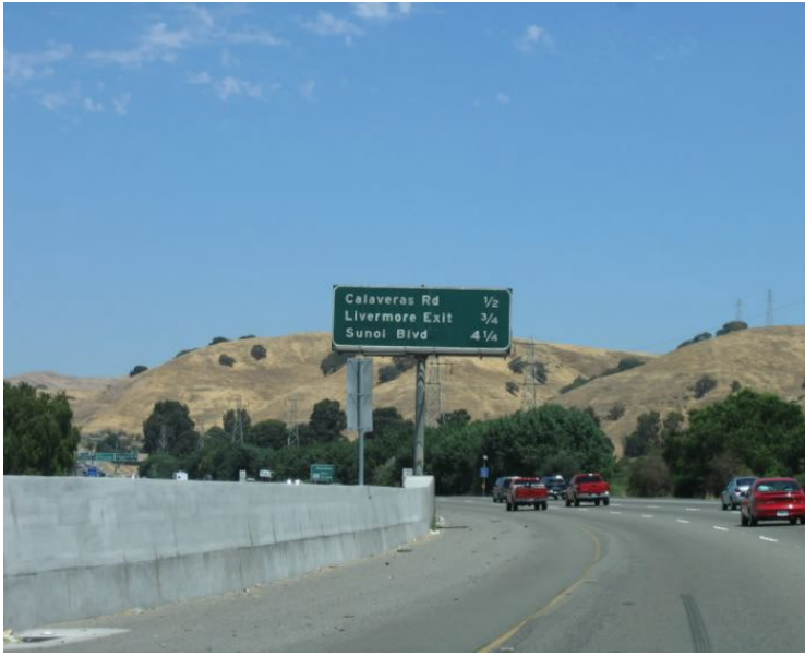
I-680 northbound approaching the Calaveras Road off-ramp.
