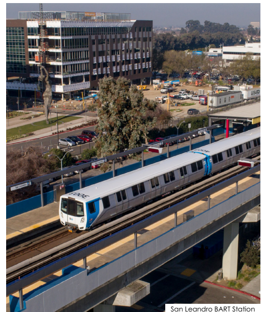
San Leandro BART Station
