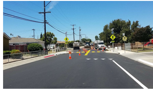
City of San Leandro – Pavement Rehabilitation Program (Brown Ct.)
