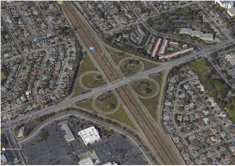
Current interchange at I-880/Winton Avenue.
