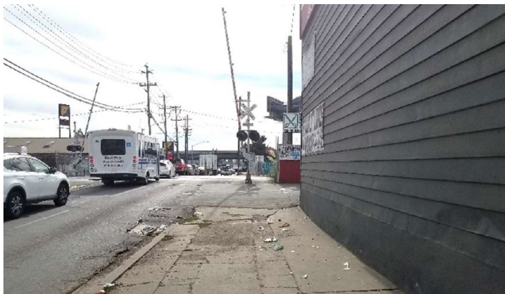
Southwest approach to the rail crossing along High Street in the City of Oakland.
