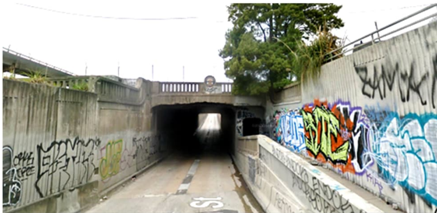
7th Street, approaching Union Pacific Railroad bridge from the east.
