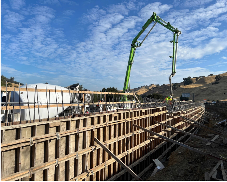
Work on the new I-680 median.
